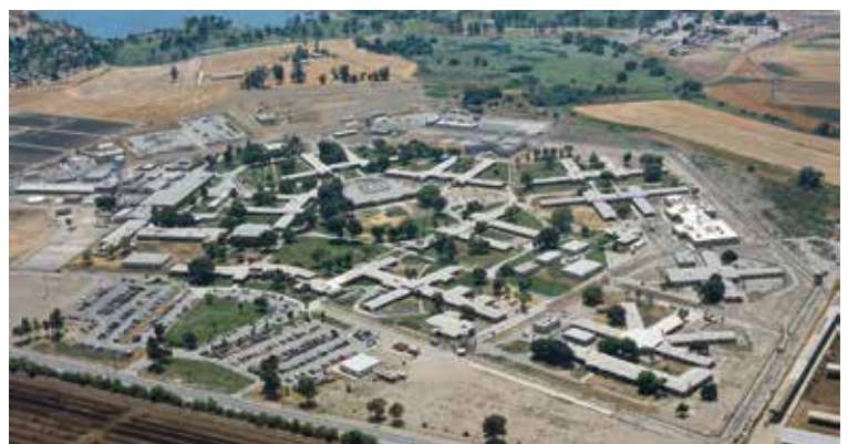
Red-Tagged facilities RJD in San Diego, CA (left) and CIW in Chino, CA (right)
